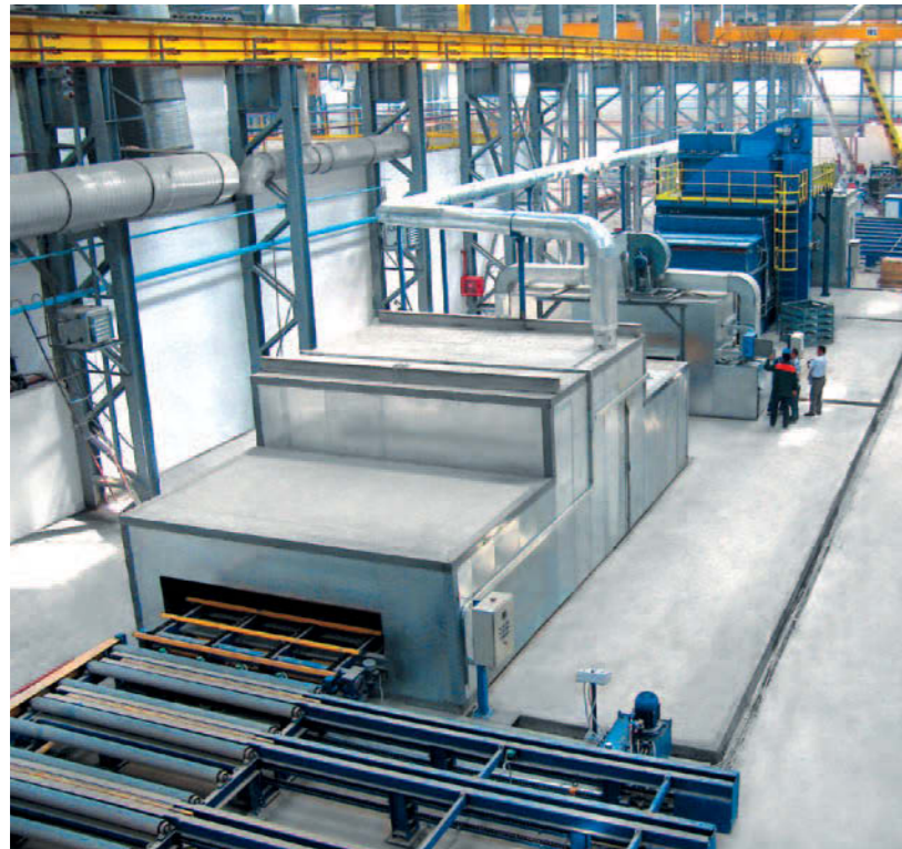
Shot blasting and preservation line for metal roll
